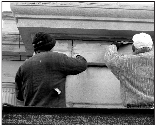
Masons grinding out and tuckpointing damaged joints. (Photo by Fred Zahn)
